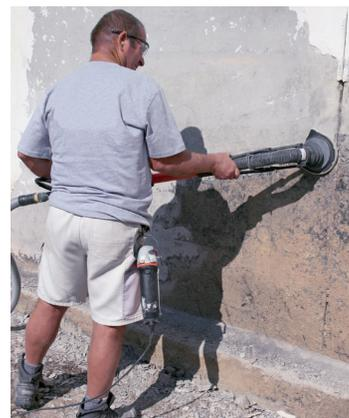
Grinding bitumen coating with PCD grinding disc
